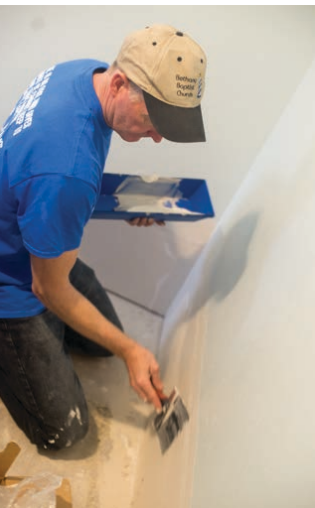
Herb Seidler mudds drywall in a flood-damaged home.
